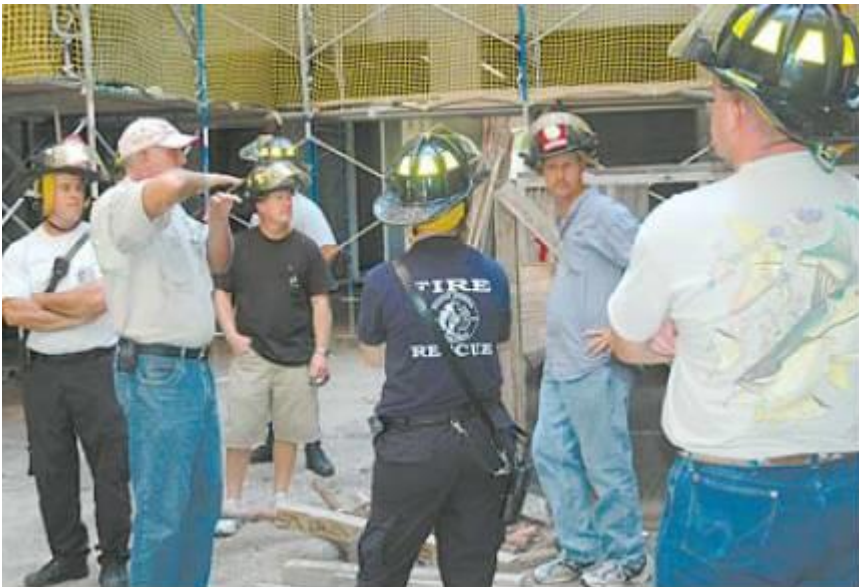
Punta Gorda Construction Management Construction Superintendent Doug Quick goes over a construction detail with a class of Punta Gorda firefighters.
