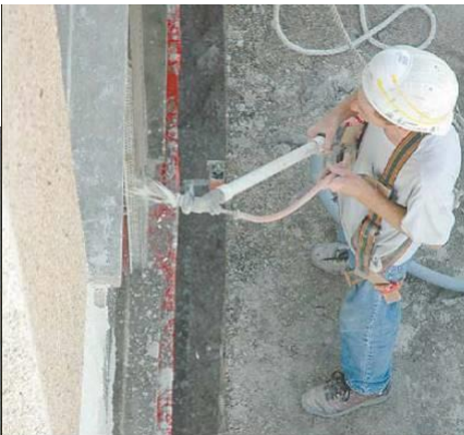
Above, a worker blows on the wet final coat, which is then troweled and blown with shell from this blower/hopper combination, below.
